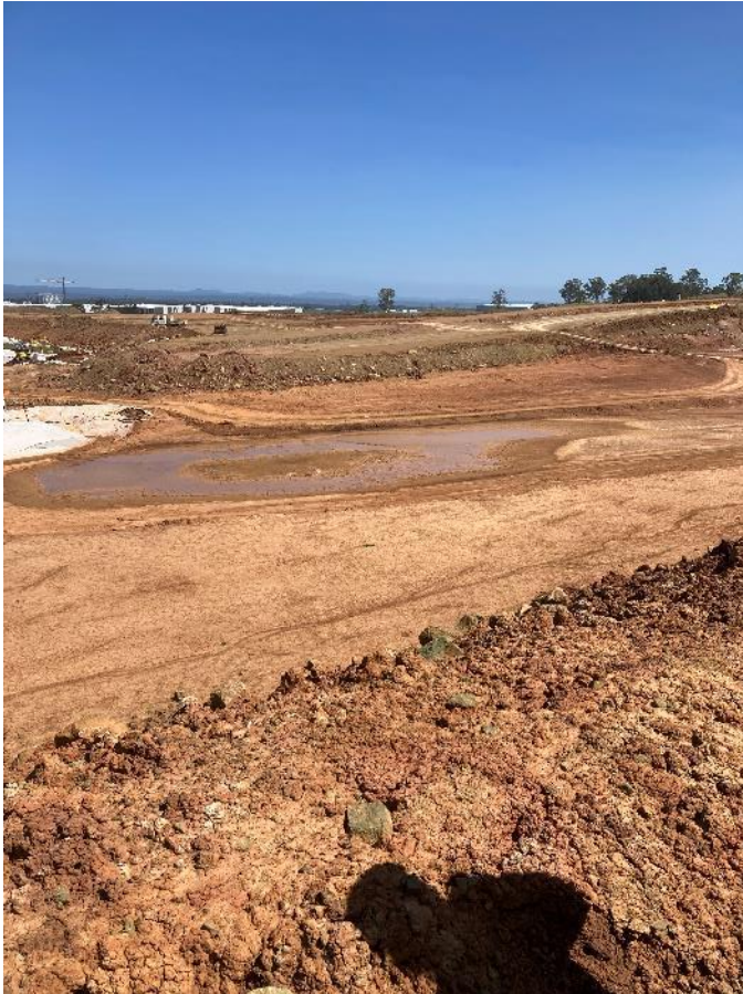
Photo 3: Construction Area, 7 February 2025
